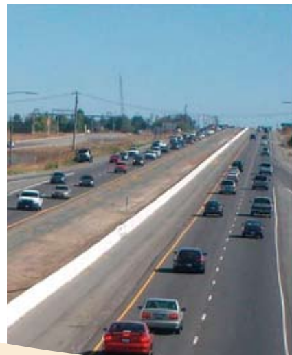
I-215 Widening Project in Murrieta
